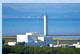
[Administrative facility] Kita Ishikari Sanitation Center
